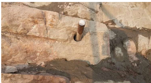
Figure 5: Centralizers at the outer end of nail
