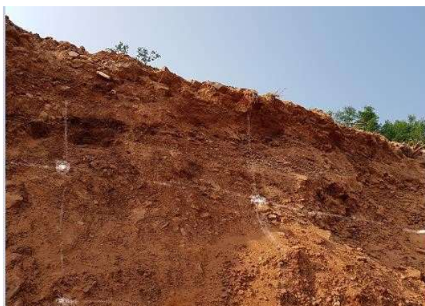
Figure 1: Marking of drill locations on the slope
